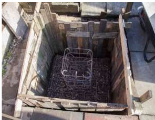
Pier foundation ready for concrete
