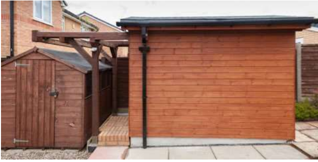
Finished observatory showing the roof closed
