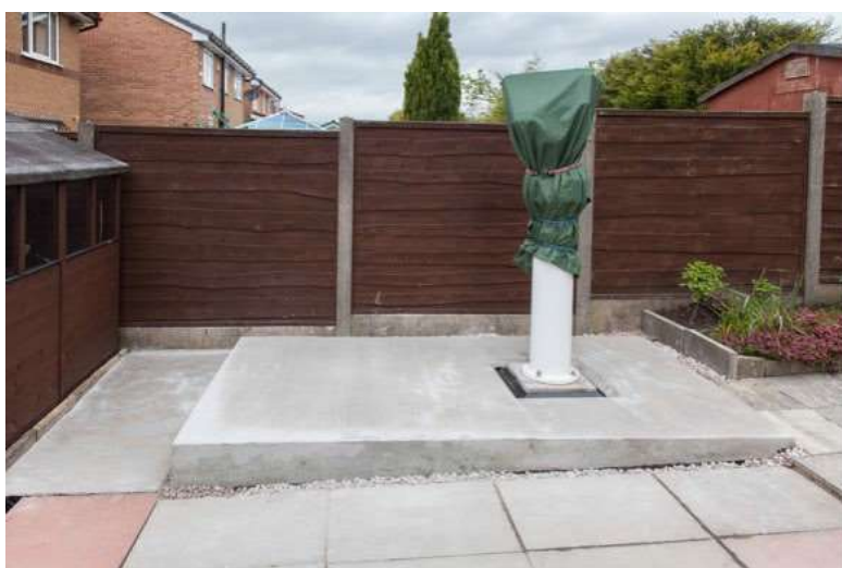
Concrete base for the observatory.
