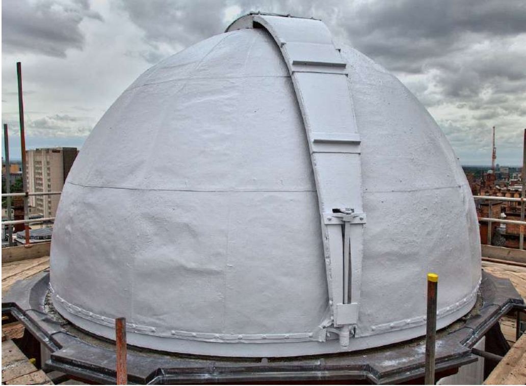
Dome after refurbishment
